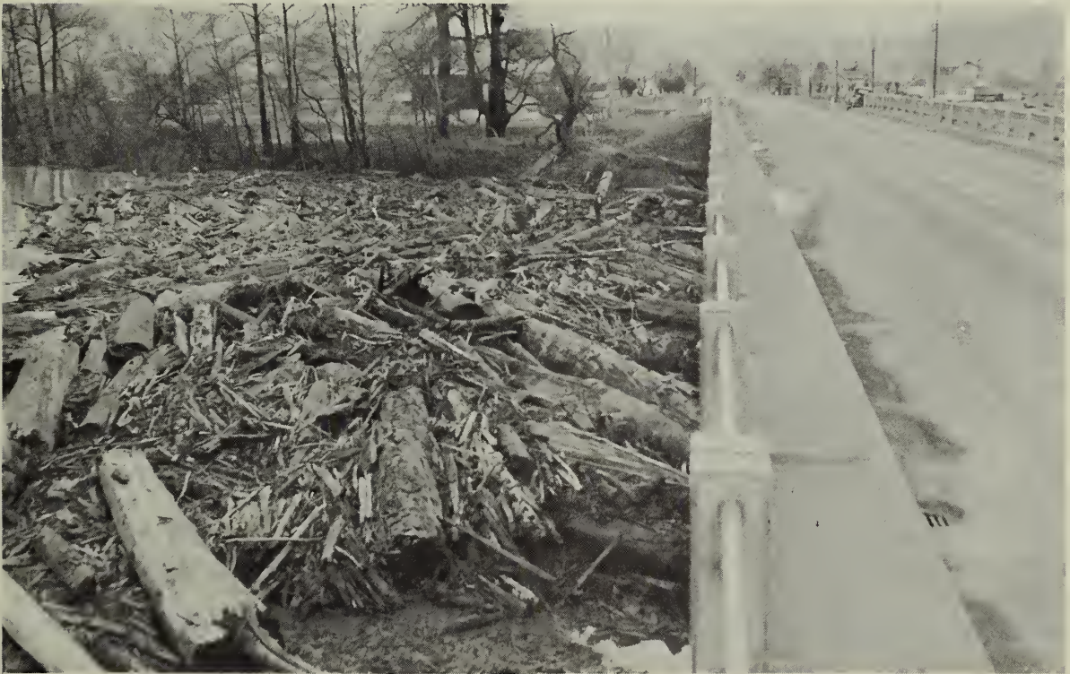
Photo 27.--Debris against U. S. Highway 101 bridge must be removed before the bridge is damaged, Trask River, Oregon, 1956. SCS photo.
